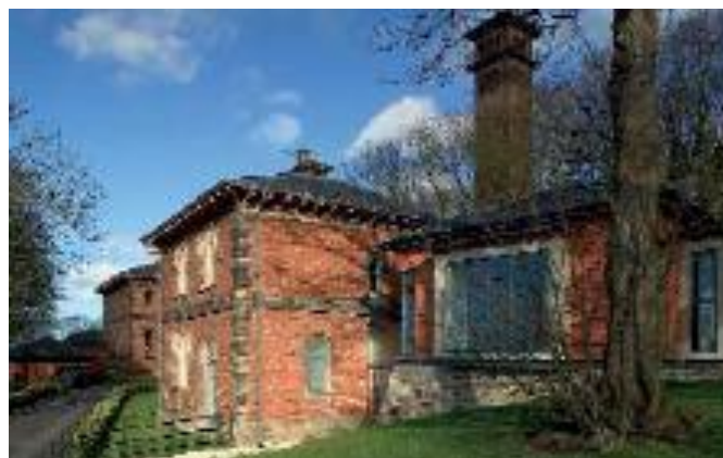
The sympathetic water tower conversion development adjacent
